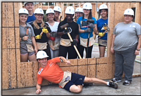
Habitat For Humanity Wall Raising
